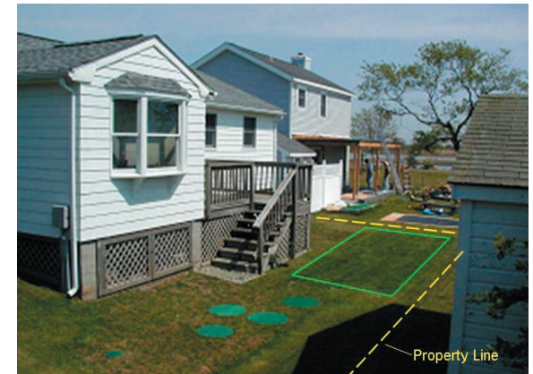
Shallow narrow drainfield following a recirculating media filter. The drainfield is visible as the area with greener lawn, also showing additional nutrient uptake by plants. In this area, the drainfield helps protect local drinking water wells and coastal pond water quality.
