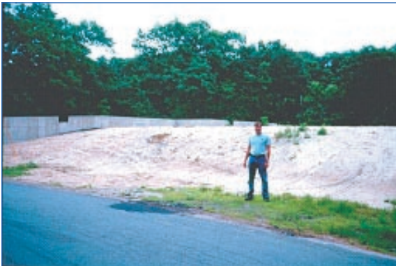
Mounds or fill systems can be 5-6 feet high, affecting the use of a property and changing the character of neighborhoods. Runoff diverted to nearby properties is often a serious problem on wet sites.
