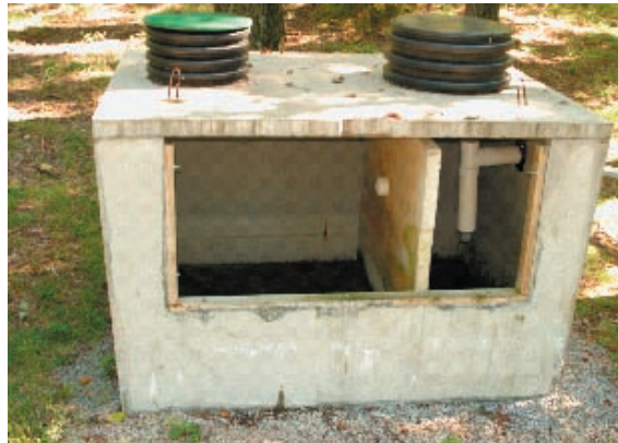
A double-compartment septic tank is more efficient in trapping solids than the standard single-compartment tank and may be required under local, county or state regulations. These are commonly used with advanced treatment systems, where the second compartment may double as a pump chamber.
