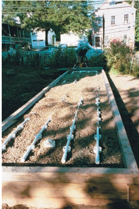
Raised bottomless sand filters, following a recirculating media filter. The system shown below serves a single-family home, and was installed as a repair to a failed cesspool. The system on top left serves a multifamily and commercial property in a village center. The distribution lines will be covered with gravel.
