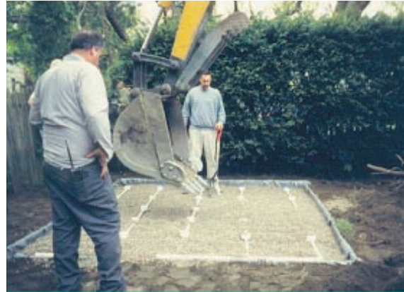
Installing a sand filter.
