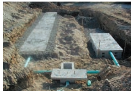
Shallow Leaching Chamber (flow diffuser)
