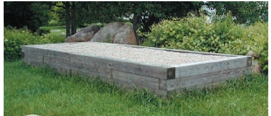
Raised bottomless sand filters, following a recirculating media filter. The system shown below serves a single-family home, and was installed as a repair to a failed cesspool. The system on top left serves a multifamily and commercial property in a village center. The distribution lines will be covered with gravel.
