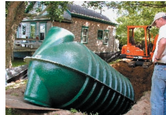
Fiberglass and PVC tanks have the advantage of being lightweight and easy to maneuver where access for heavy equipment is limited; however, these are more susceptible to damage with improper installation or maintenance.
