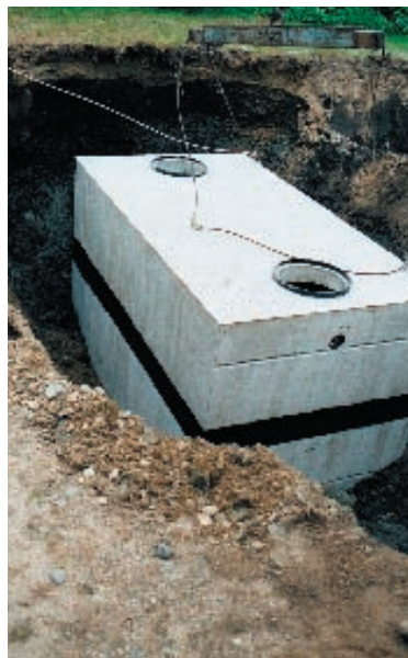
Concrete Septic Tank. Large capacity tank showing seam where tank was assembled. Testing for watertightness ensures seams are properly sealed.
