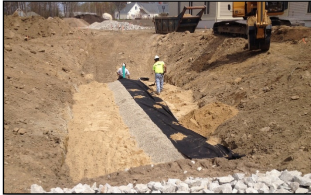
BIO-RETENTION DRAINAGE SYSTEM INSTALLATION
