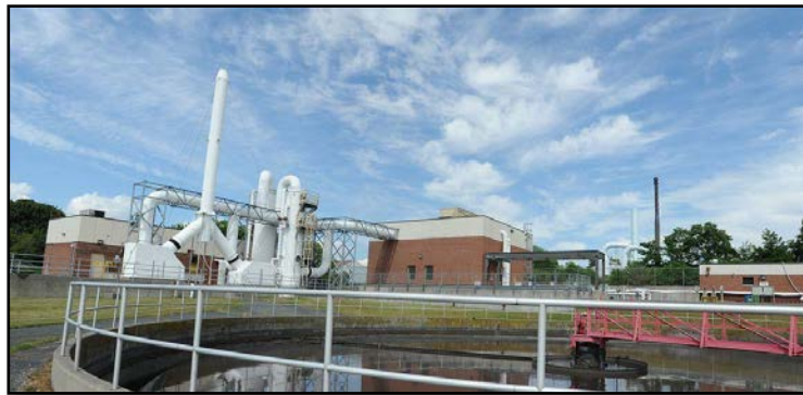
FALL RIVER WASTEWATER TREATMENT PLANT
