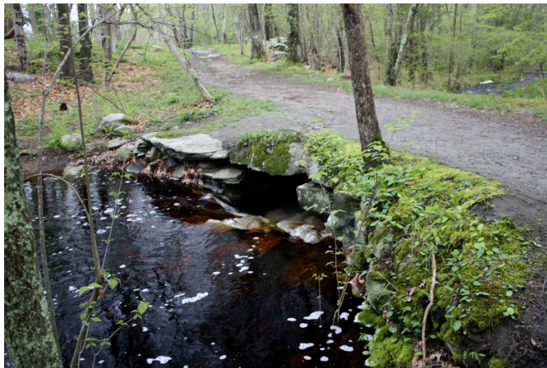
SLAB BRIDGE ON EIGHT ROD WAY IN WEETAMOO WOODS
