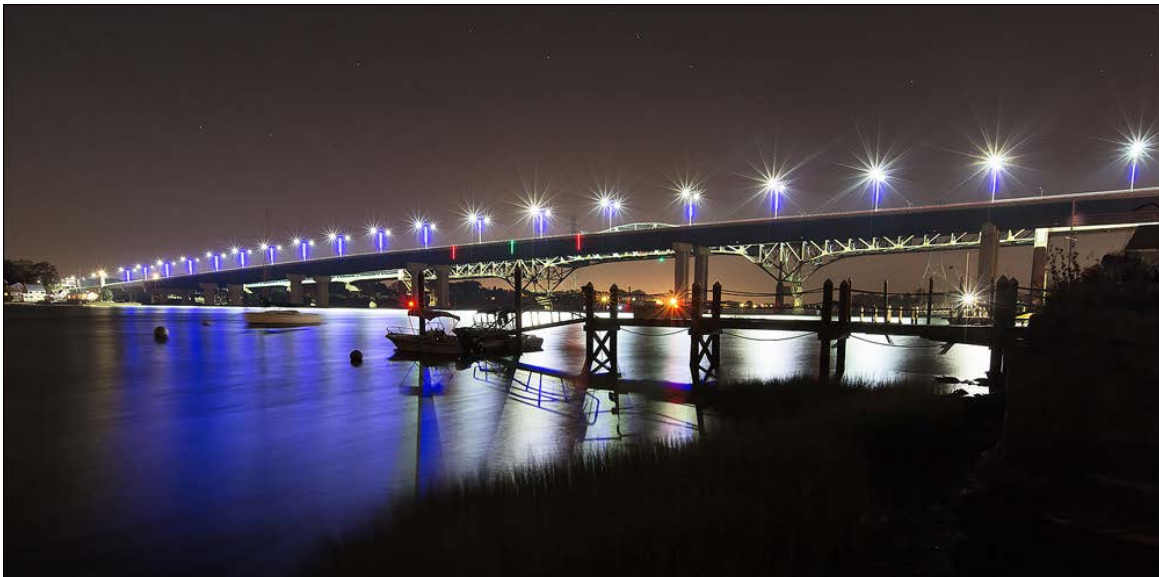
SAKONNET RIVER BRIDGE
