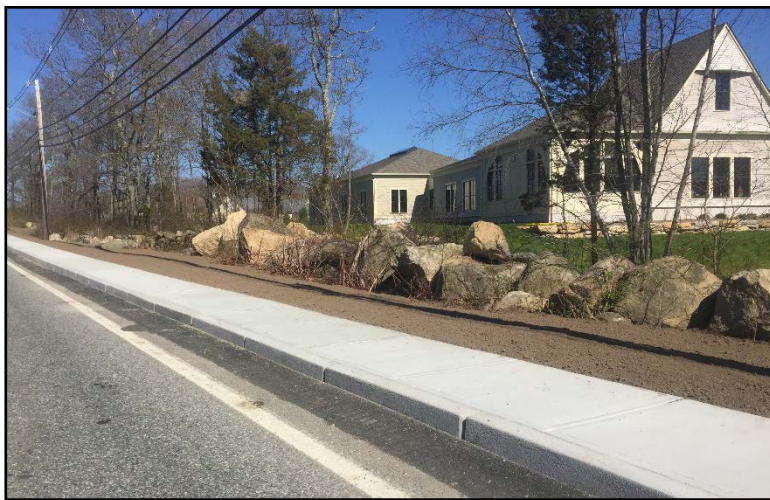
NEW SIDEWALK ALONG BULGARMARSH ROAD
