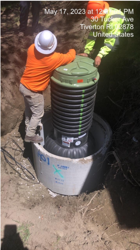
Figure 2 Grinder pump installation.
